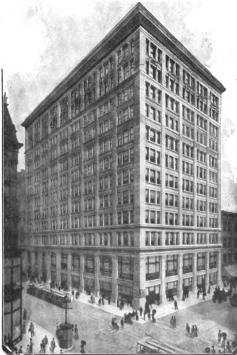
MERCHANTS' LOAN AND TRUST BUILDING, Northwest Corner Adams and Clark streets, Chicago.
