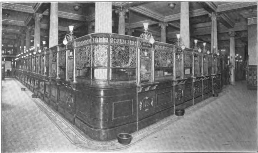
MAIN BANKING ROOM.
