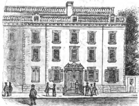
THE WALTON HOUSE, LOCATED IN FRANKLIN SQUARE, PEARL STREET, IN WHICH THE BANK OF NEW YORK COMMENCED BUSINESS JUNE 9, 1784.
