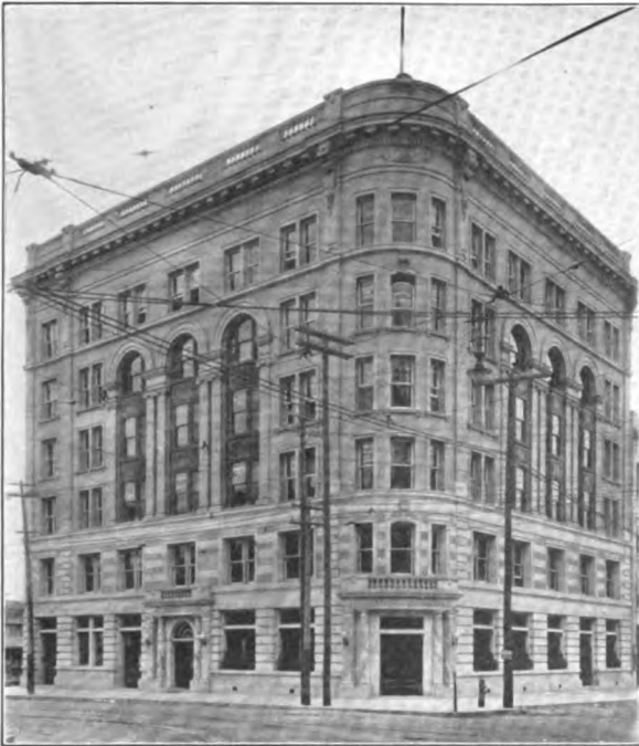
COMMERCIAL NATIONAL BANK BUILDING.
