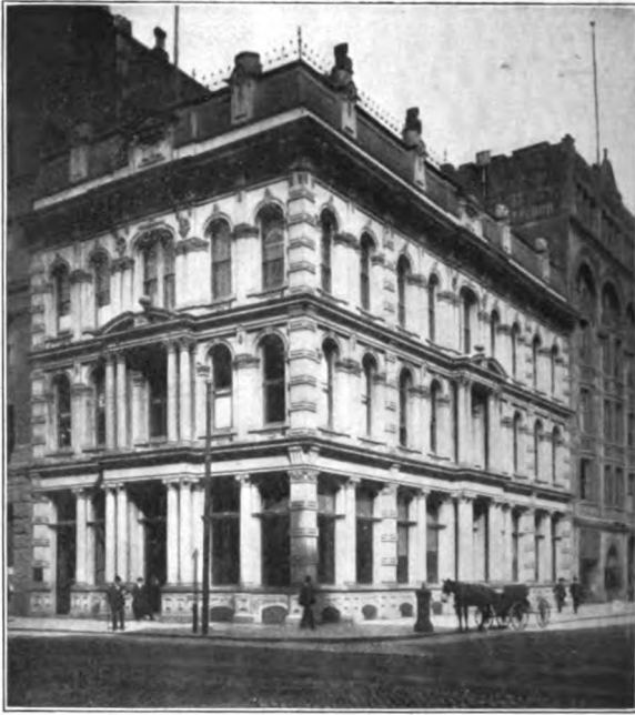
ANGLO-CALIFORNIAN BANK, LIMITED. Building destroyed. Temporary office, southwest corner Clay and Franklin Streets.
