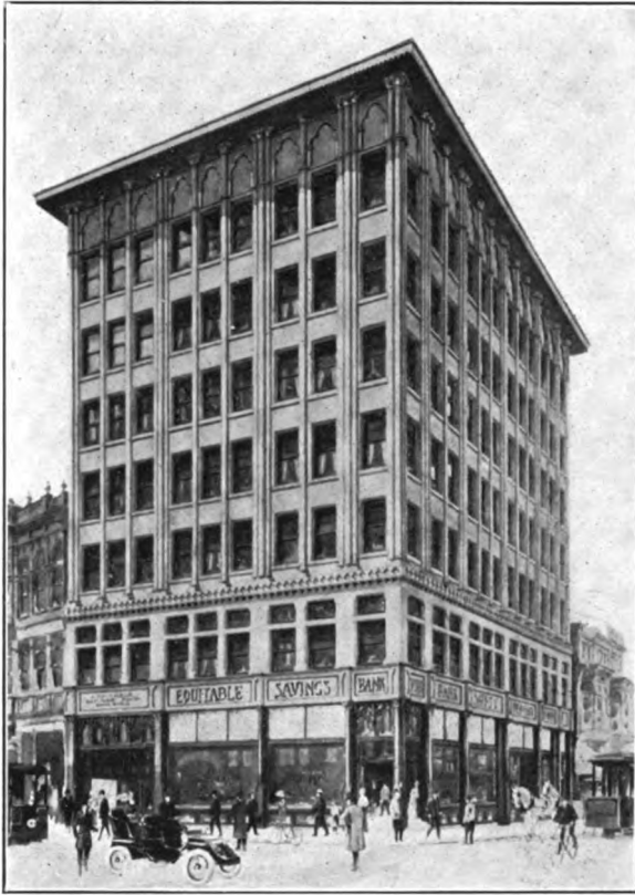
EQUITABLE SAVINGS BANK. (Under Construction.)
