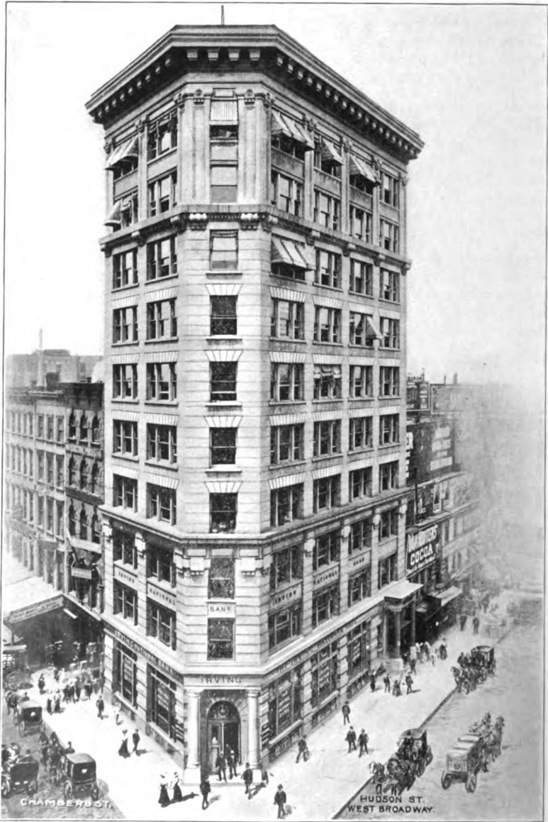
IRVING NATIONAL BANK BUILDING, NEW YORK.
