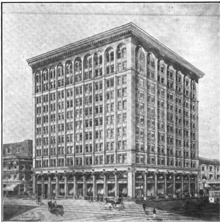
SECURITY SAVINGS BANK BUILDING, (Under Construction.)
