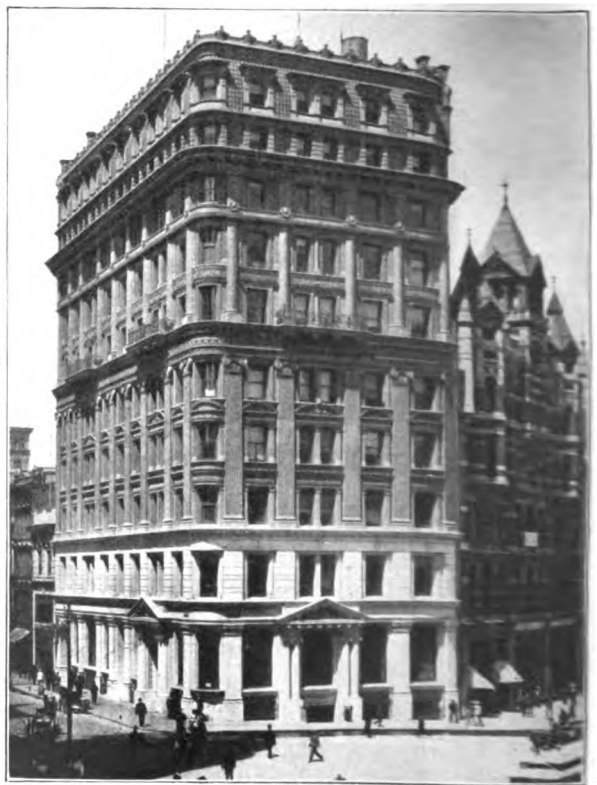
UNION TRUST COMPANY. Building damaged, but available for use.
