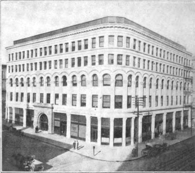
GERMANIA NATIONAL BANK. Building destroyed. Temporary office, 21 1/2 Laguna Street.
