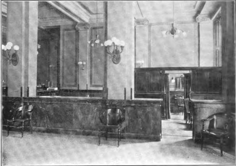
VIEW OF WOMEN'S ROOM.
