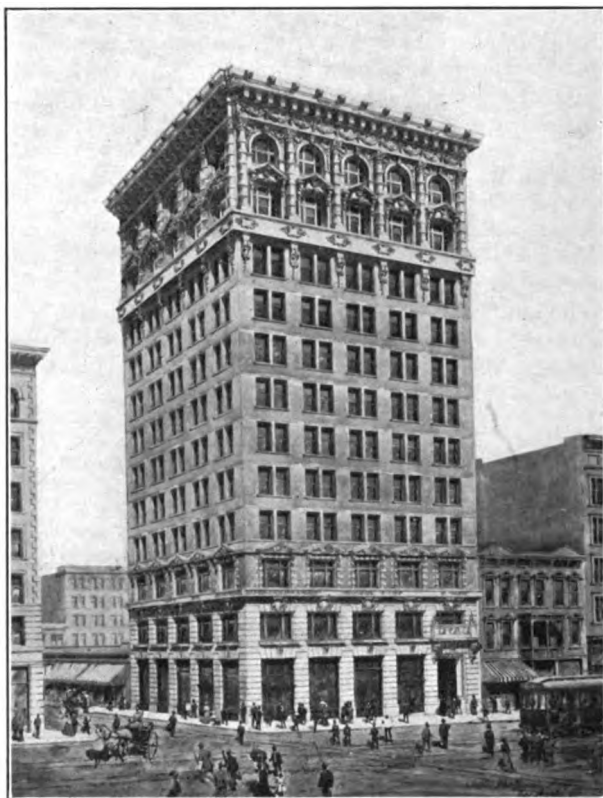
UNION TRUST BUILDING. (Home of Southern California Savings Bank.)
