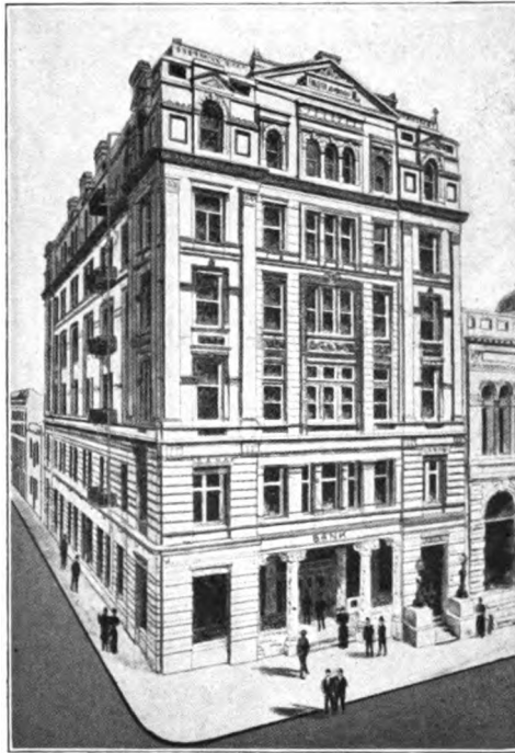
SAN FRANCISCO SAVINGS UNION. Building destroyed. Temporary office, 2617 Pacific Avenue.
