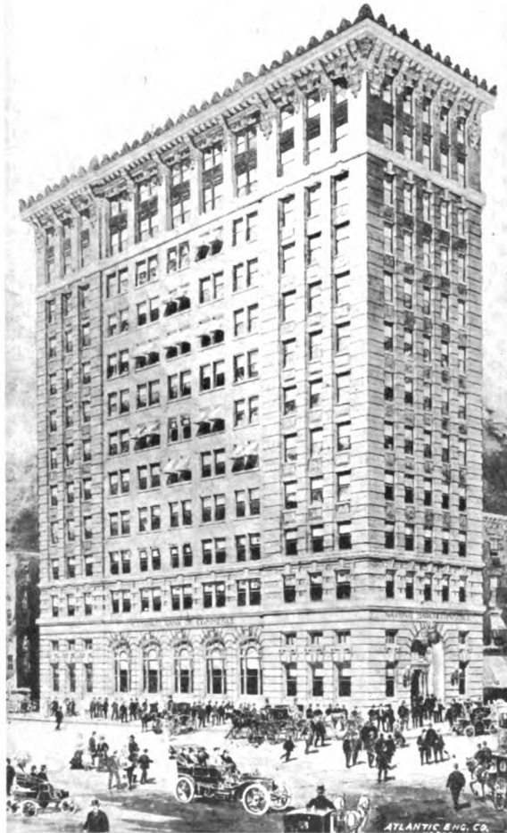
NATIONAL BANK OF COMMERCE BUILDING, NORFOLK, VA.
