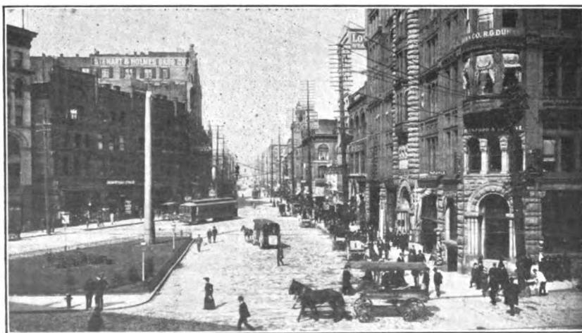
VIEW ON FIRST AVENUE.
