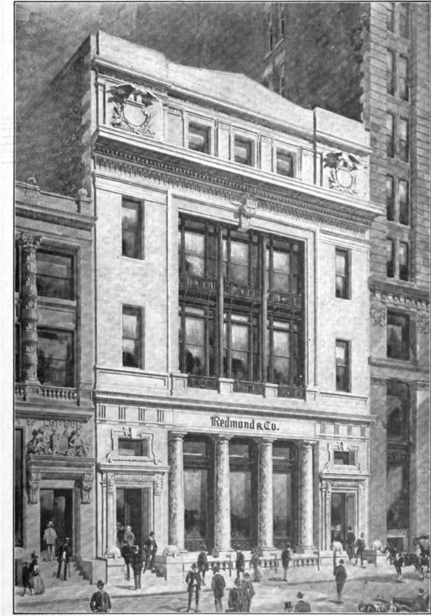
THE REDMOND & CO. BUILDING.
