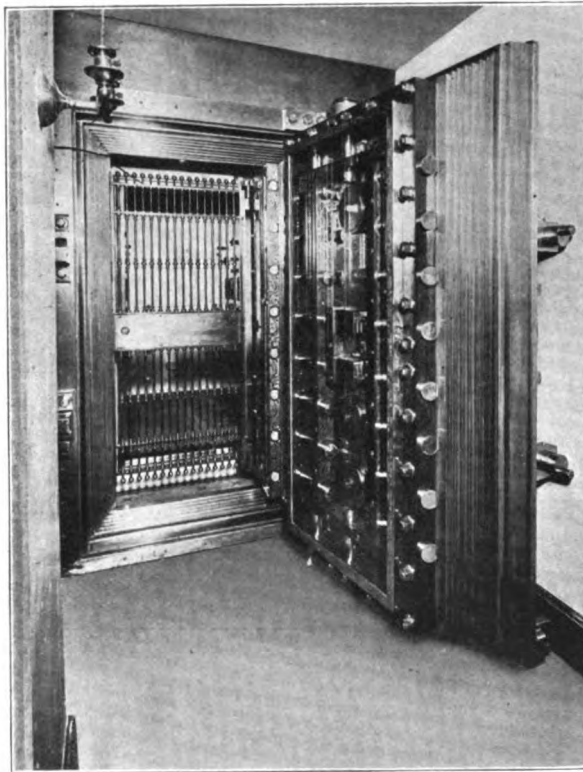
The Vault. MERCANTILE NATIONAL BANK.
