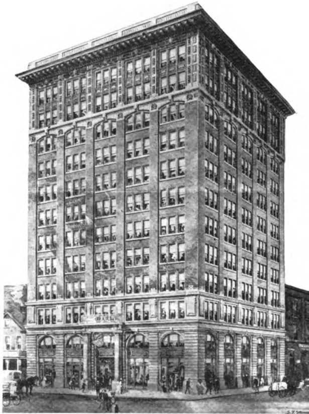
THE WELLS-FARGO BUILDING.
