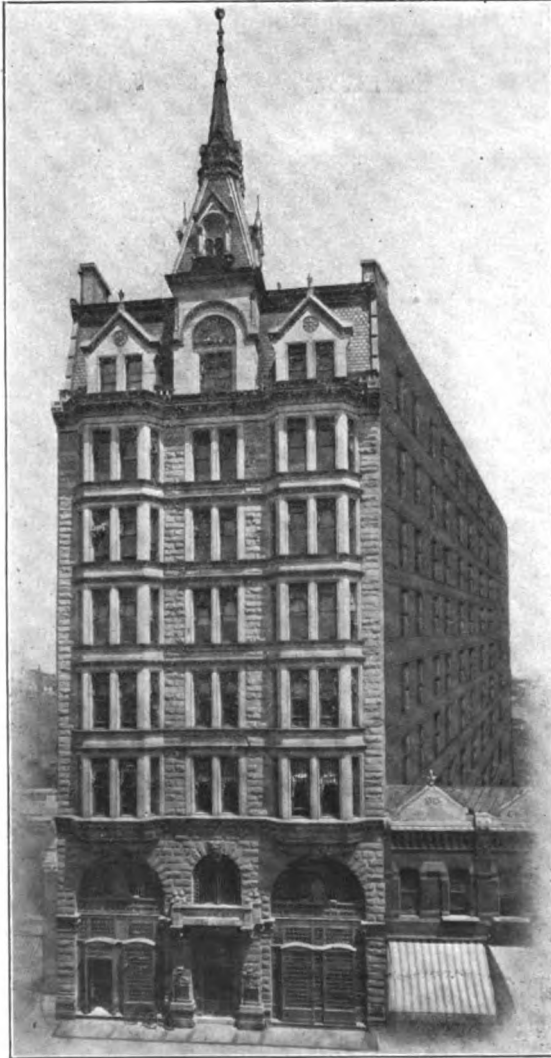
AMERICAN NATIONAL BANK BUILDING, WASHINGTON.
