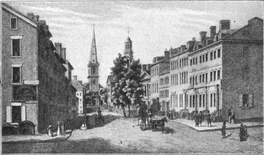
WALL STREET IN 1825, LOOKING WEST FROM WILLIAM STREET.
