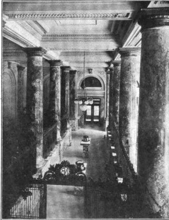
ANOTHER VIEW OF BANKING ROOM.
